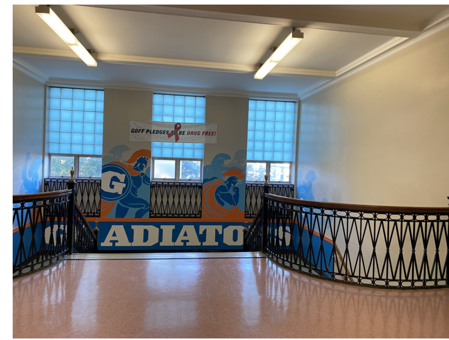
EXISTING SECOND FLOOR RAILING
